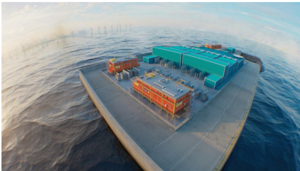
Figure 2 PEZ Energy Island (Belgium)
